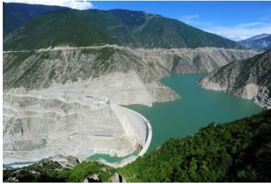
Figure 7. Deriner Dam in Artvin [2]
