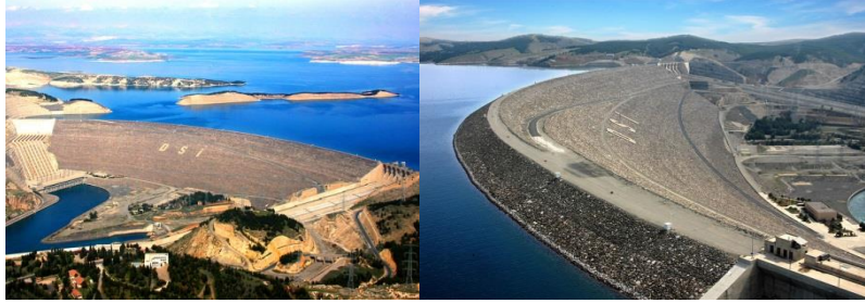
Figure 4. Atatürk Dam in Adıyaman / Şanlıurfa [15]
