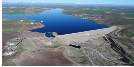
Figure 5. Pamukçay Dam in Diyarbakır [25]
