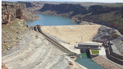
Figure 3. Dicle Dam in Diyarbakır [19]
