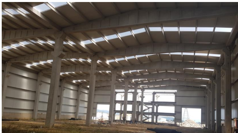
Fig.1 The general view of a typical single story precast industrial RC-building
